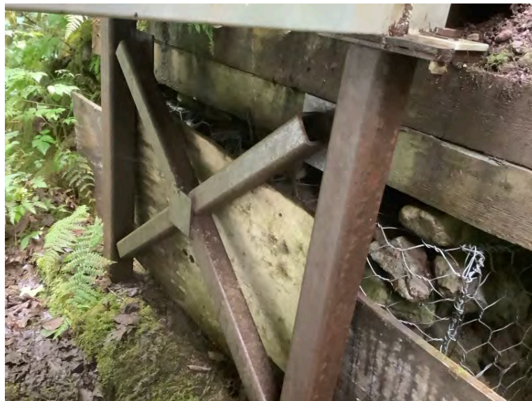
Right Bank Abutment when facing downstream
