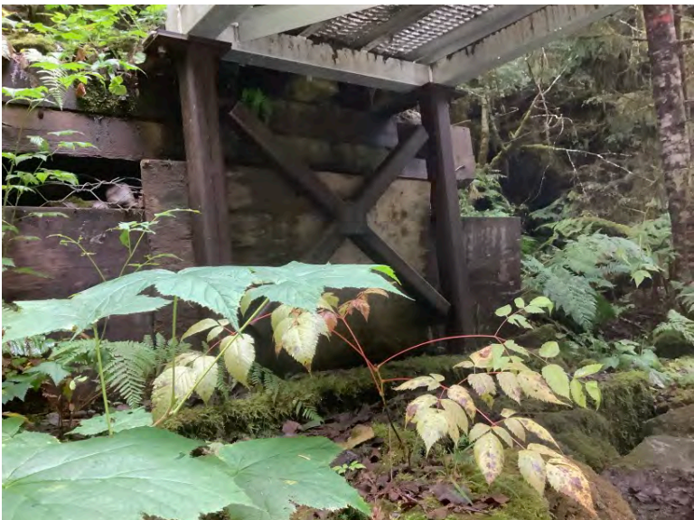
Left Bank Abutment when facing downstream
