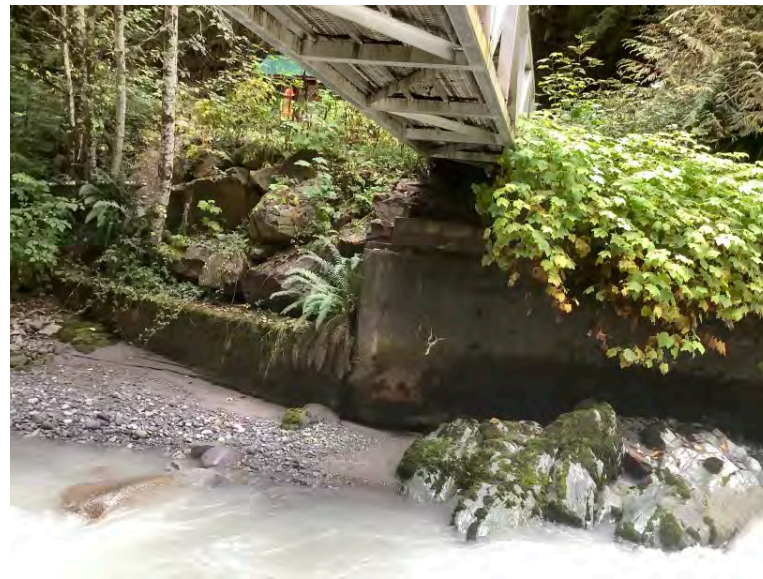
Right Bank Abutment when facing downstream
