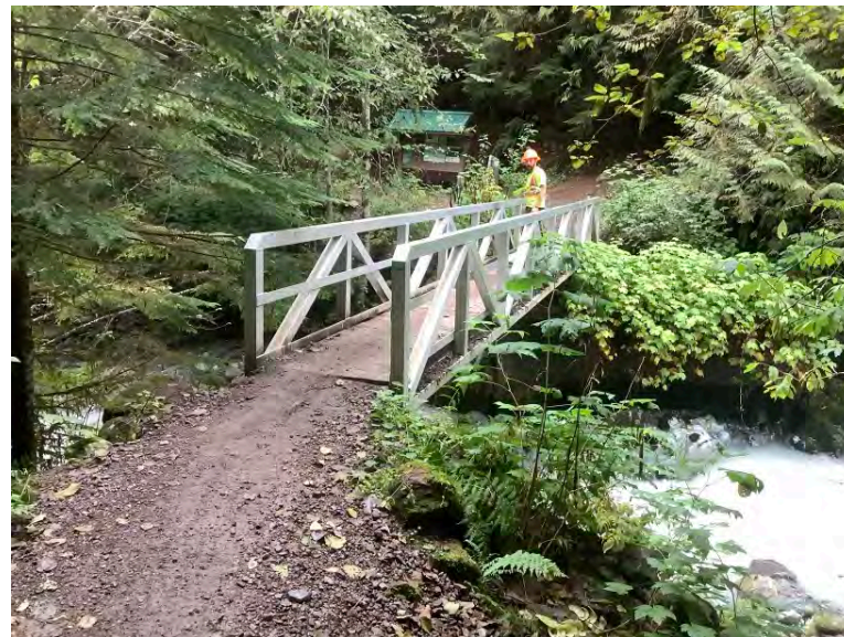
Left Bank Abutment when facing downstream
